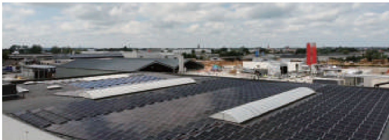
C&I rooftop project in Belgium, Europe
