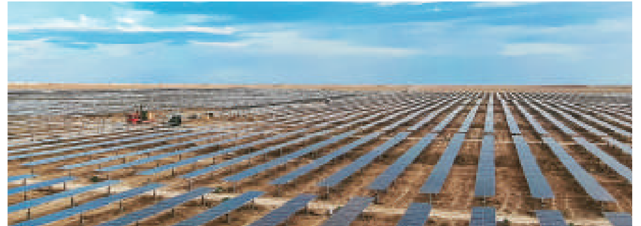
Ground-mounted power station project in Qinghai Province
