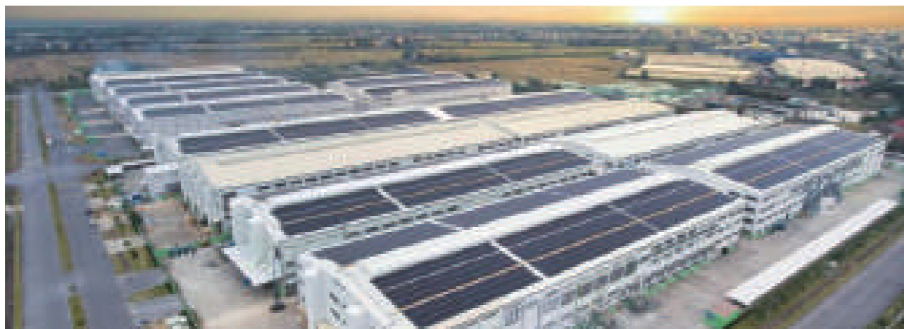
Distributed Project in Vietnam
