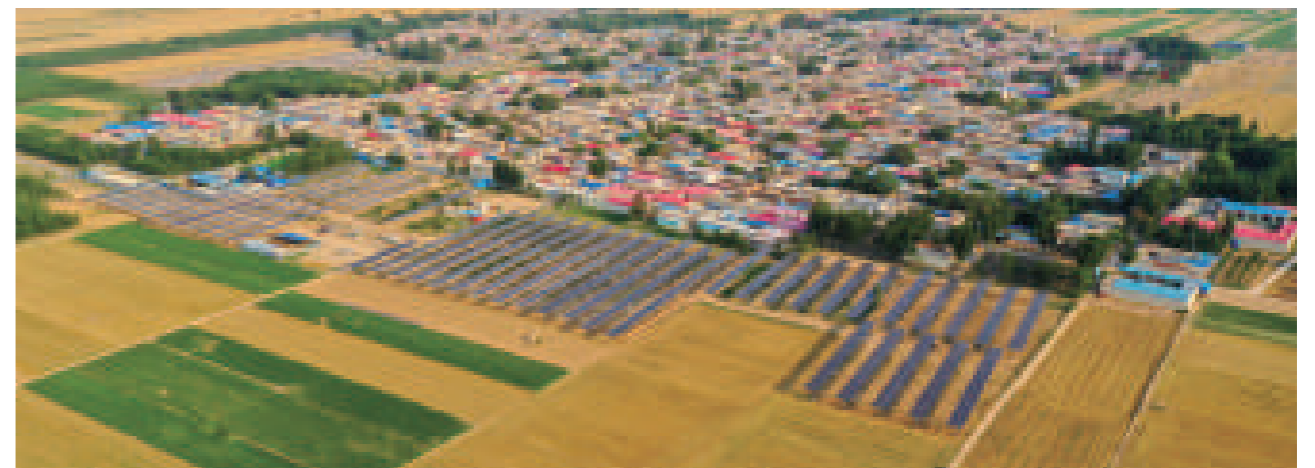
Tracker power station in Hebei Province
